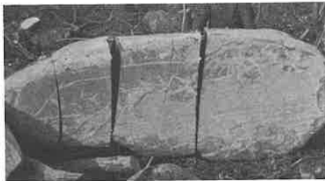
Large rock "sliced" with hydraulic splitter.
