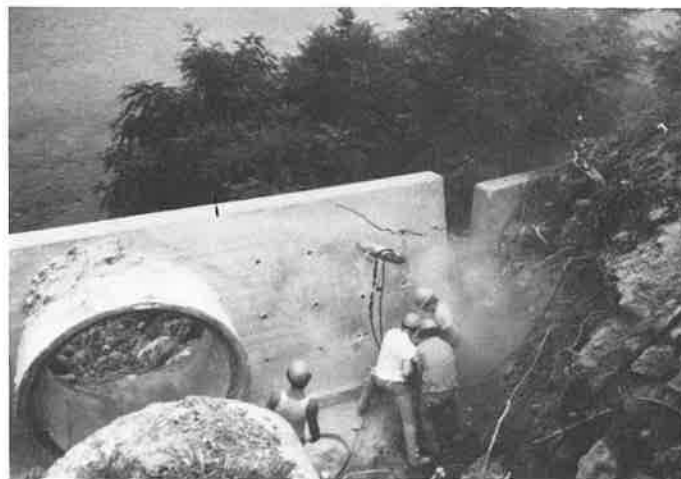
Culvert wall broken in seconds with hydraulic splitter.
