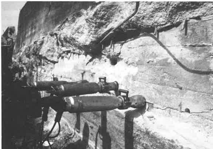
Use of two or more splitters can quickly double or triple the breaking force on massive sections of concrete or rock. The above shows three splitters breaking a 10' concrete wall in a few seconds.
