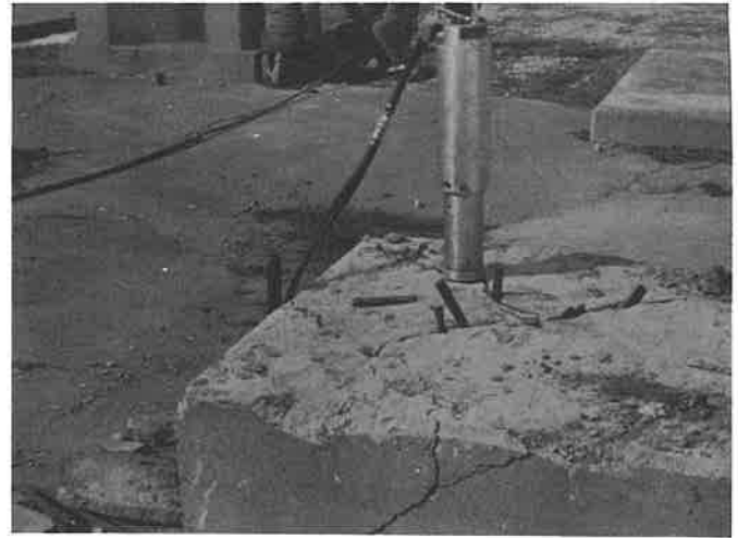
Reinforced concrete broken with hydraulic splitter.
