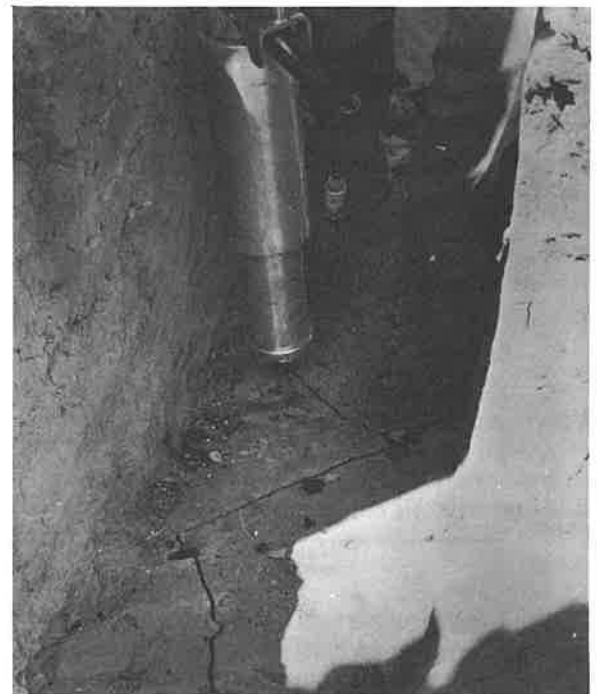
Splitter breaking rock in small trench.
