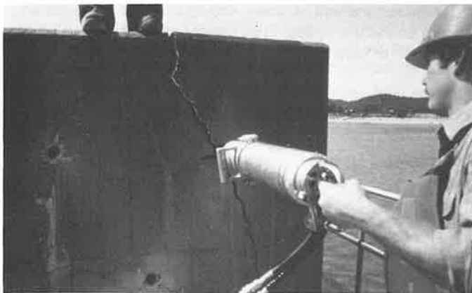
Concrete being removed on Ohio River Dam.
