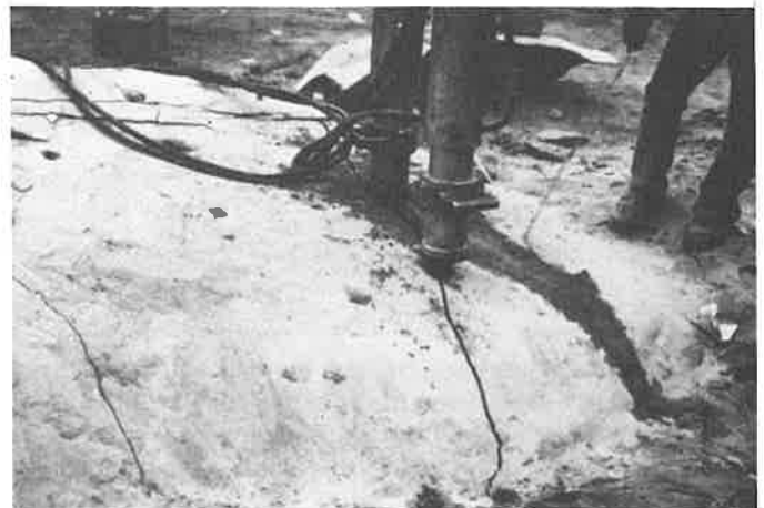
Two hydraulic splitters break submerged boulder 15' across, 12' deep and 20' long.
