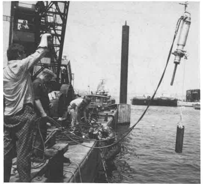
Hydraulic Splitter is lowered into New York's East River for underwater operation.
